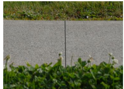
Smooth Sidewalk surface with Sawcut Contraction Joint
