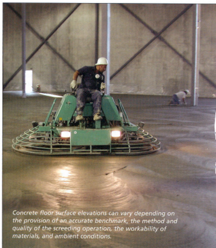
Concrete floor tolerances must provide designers with definitive practical limitations for their calculations and contractors with clear-cut performance criteria. However, they commonly go uninspected until something goes wrong.
